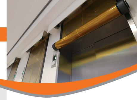
Codes and Standards. The M600 works in conjunction with the already fire-rated elevator doors to exceed the NFPA and IBC requirements for a smoke- and draft-control assembly. This enables the elevator to open directly onto the corridor, eliminating the need for additional doors at the elevator constructed lobby space.
